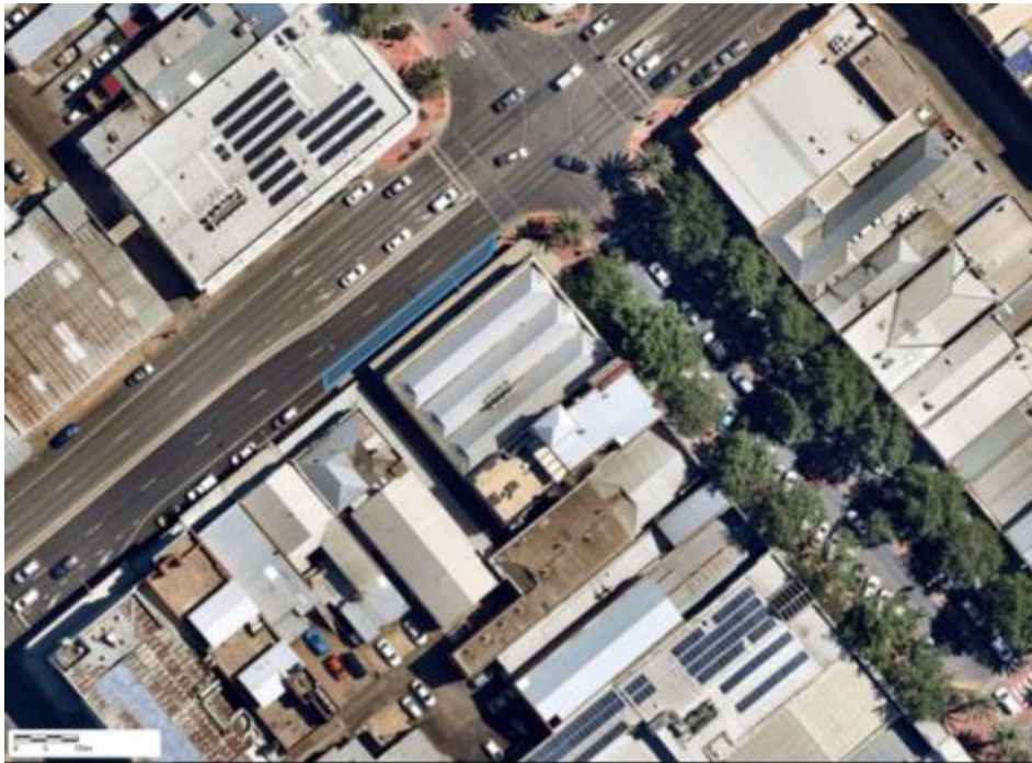
Figure 6. Location of bus stop on Brisbane Street
